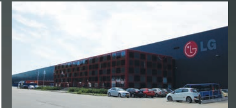
European Air Conditioning Distribution Center
